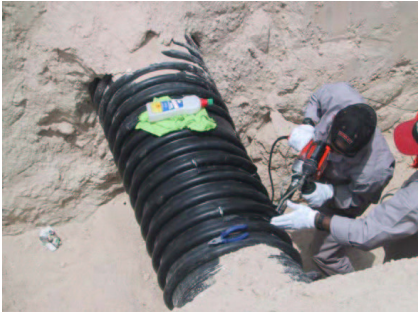
Figure 5: Extrusion welding of the pipe piece
