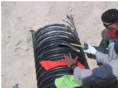
Figure 2: Removal of the core tube
