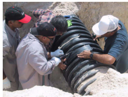
Figure 4: Place a solid wall pipe piece on the spot
