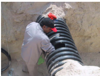
Figure 3: Clean cutting edges
