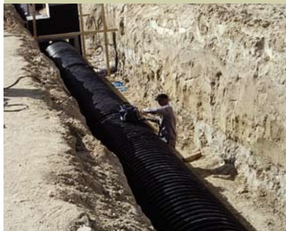
Installation of a sewage pipe with a complete manhole
