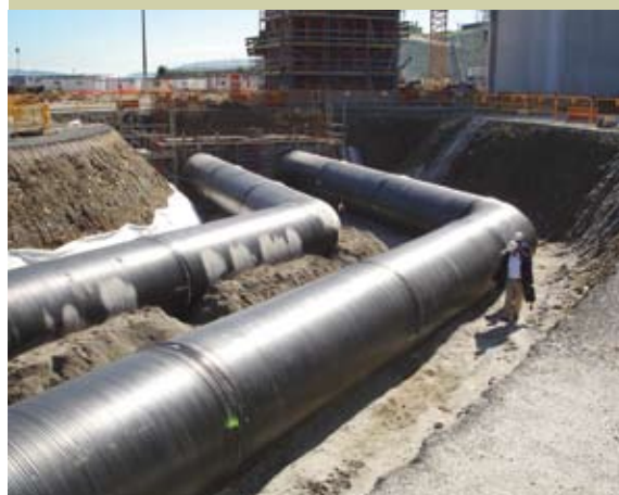
Installation of a TWIN-pipe DN/ID 2000 mm with fittings
