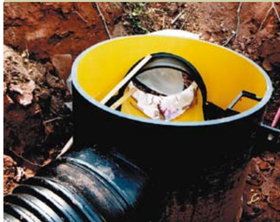
Standard manhole DN/ID 1000mm
