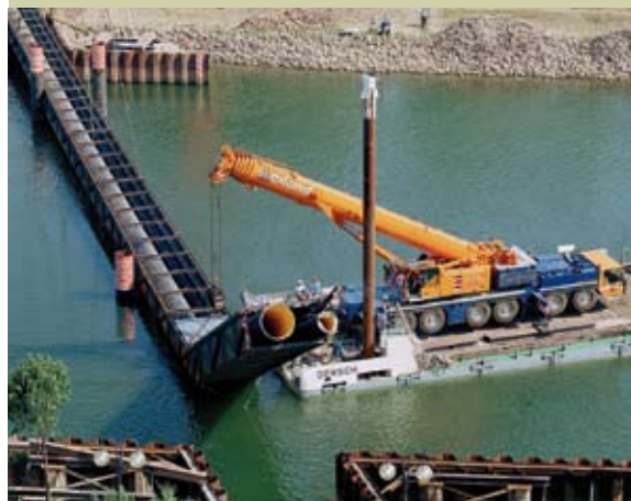
Siphon pipe – installed in a river
