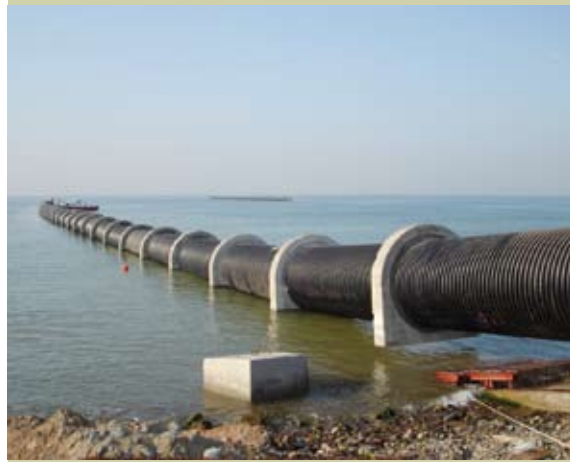
Sea outfall pipe line DN/ID 1800 mm
