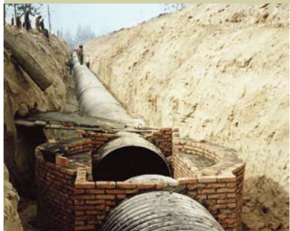
Krah pipe with a manhole - produced with bricks
