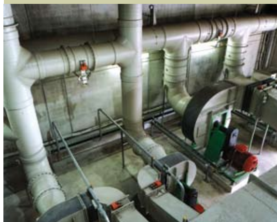
Industrial ventilation pipes
