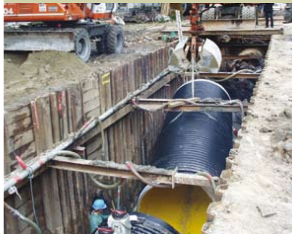
Sewer pipeline DN/ID 2000 mm
