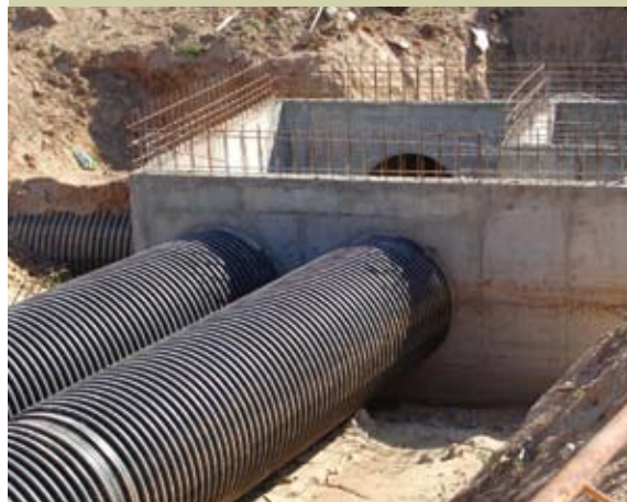
Main collector of a sewage treatment plant
