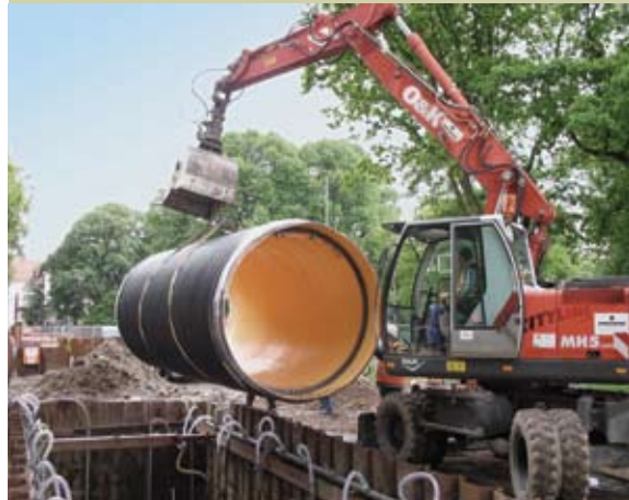
Installation of a pipe
