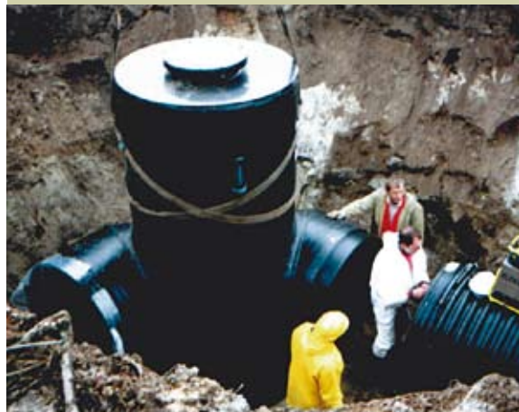
Manhole with an integrated bend and electro fusion joint
