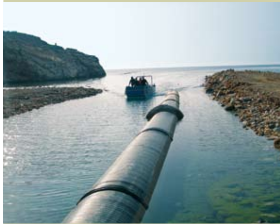
Outfall pipe line DN/ID 2000 mm
