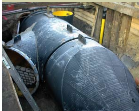
Reduction DN/ID 2400 → DN/ID 1600 mm
