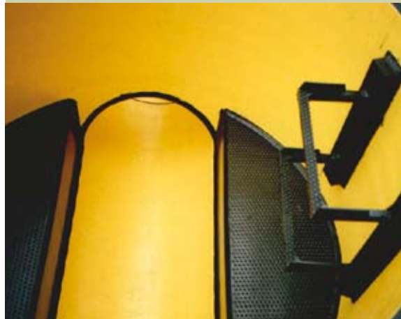
Inside of a standard manhole with a berm and stairs
