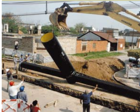
Quick manhole installation
