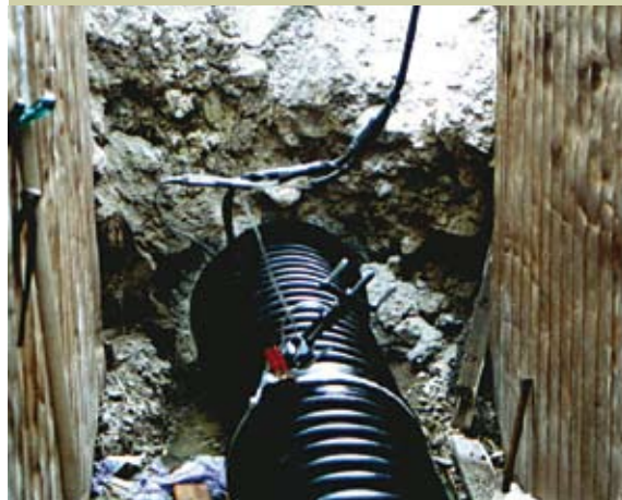
Relining of a concrete pipe
