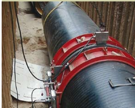
Heat element butt welding connection
