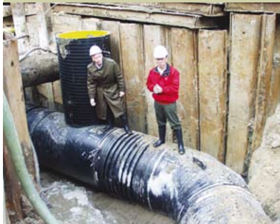
Sewer line DN/ID 1200mm with bend and manhole jointed by electro fusion
