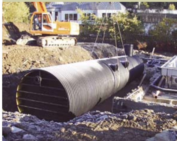
Installation of a swimming pool storage tank
