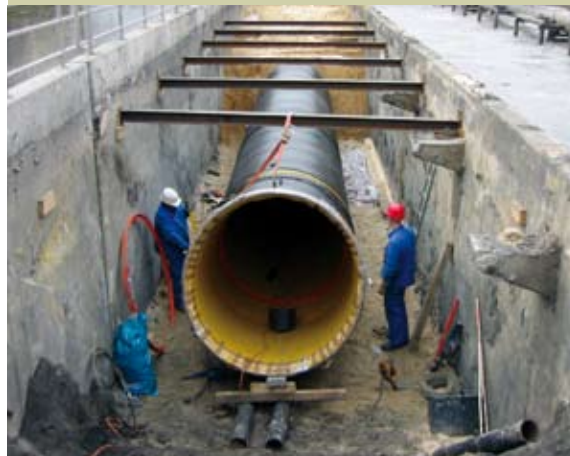
Installation of a pipe DN/ID 2000 mm
