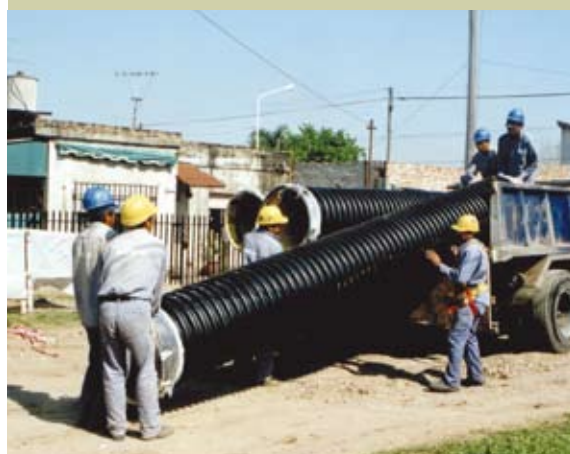
Manual unloading of a pipe DN/ID 600mm
