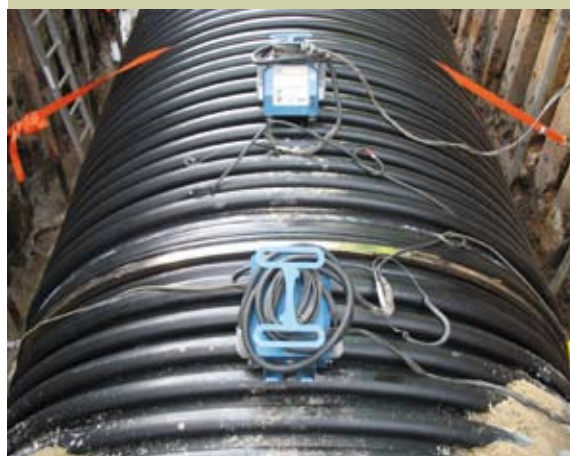
Electro fusion connection on site
