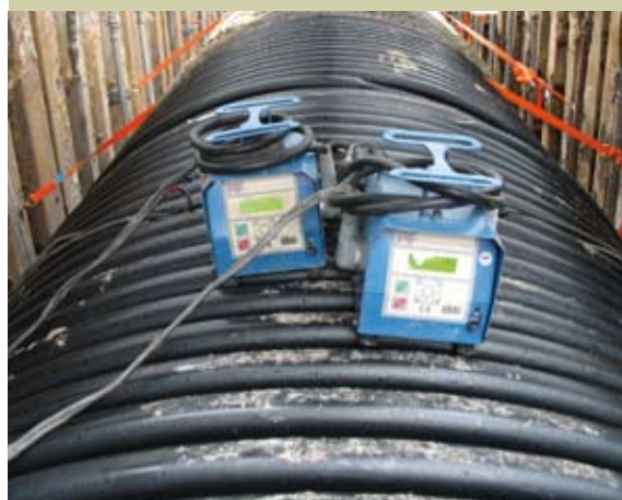
Welding of a large diameter pipe in a narrow trench
