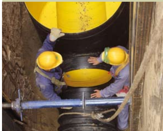
Connection of a pipe incl. manhole by the electro fusion method
