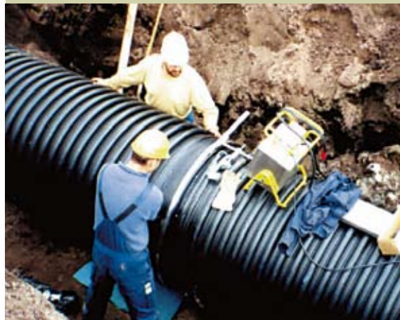
Electro fusion welding procedure
